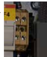
Neutral Link for total circuit isolation (control circuit)
