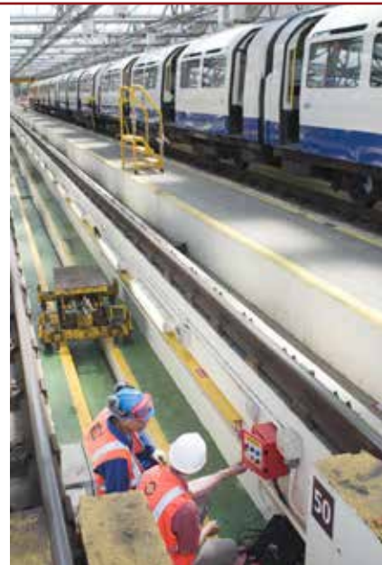
Application in Rolling Stock Repair pits
